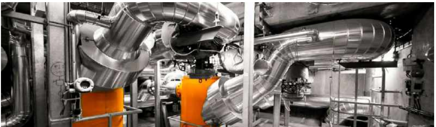
Steam transfer station; Palais Bourbon, Paris
