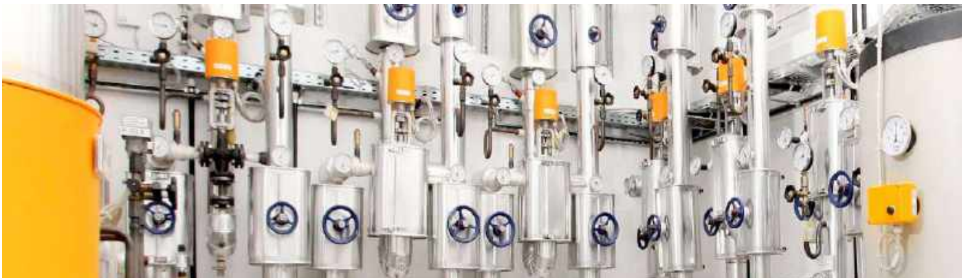
Heat transfer station with ejector heating distributor and buffer tank; Baelz head office, Heilbronn
